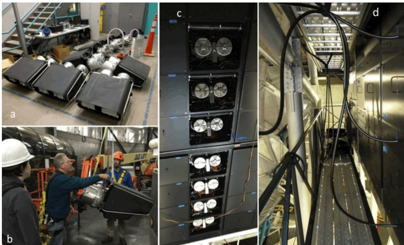
Figure 7: VIRUS spectrograph unit deployment; (a) 8 units staged for installation in HET receiving bay; (b) VIRUS unit rigged and balanced for lifting with HET dome crane; (c) 8 units installed in one of the VIRUS enclosures, prior to installation of enclosure covers; (d) IFUs installed on the other side of the enclosures, or awaiting installation after stringing from the tracker.
