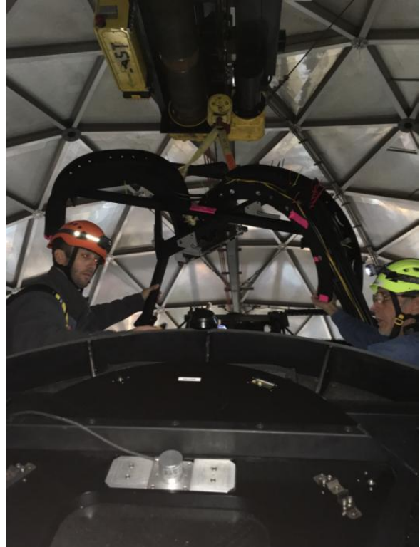
Figure 7. Left photo shows the IHMP and SR1 assembly being lifted from its mount on the focal plane assembly. Figure 8. Right photo shows IHMP and SR1 assembly suspended from dome crane
