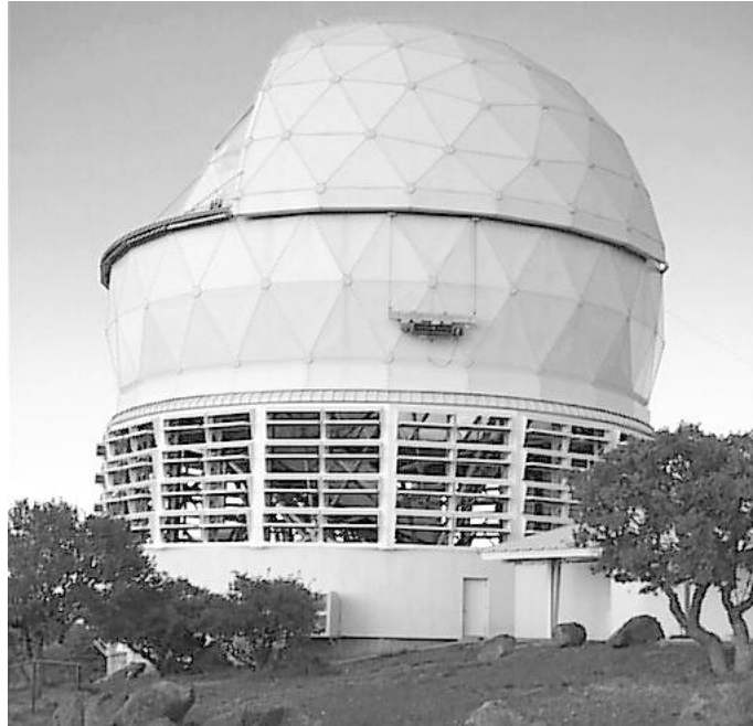
Figure 1: Western view of HET Enclosure with Ring Wall louvers and view of louver hoist.
