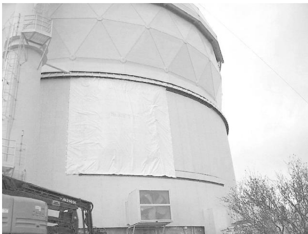
Figure 9: Weather curtain in place over opening.
