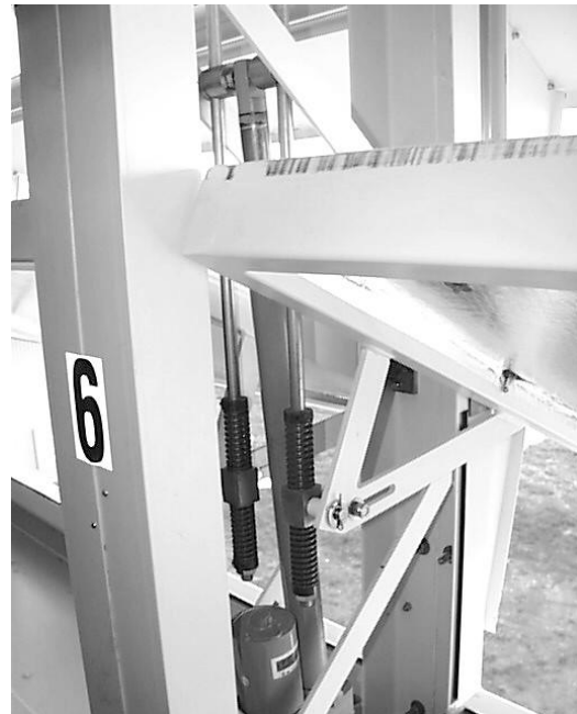
Figure 5: Detail of louver drive mechanism.
