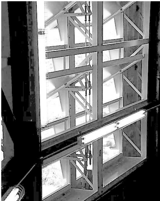
Figure 4: Interior view of louver structure.
