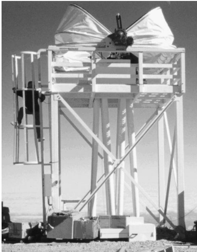
Figure 4: The ESO DIMM tower (Surrier-type truss) and platform.
