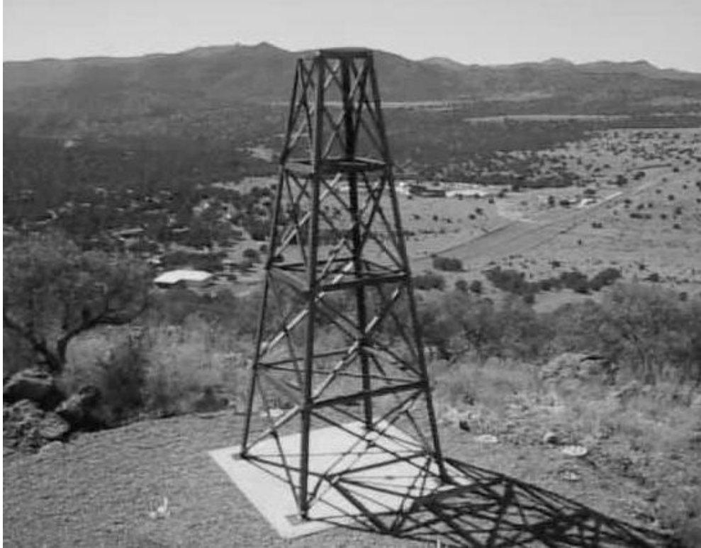
Figure 7: "Oil-Derrick" type structure prior to erection of access platform.
