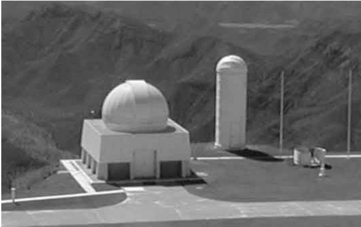
Figure 3: Gemini South's DIMM tower (right) is shielded from wind by an outer tower.
