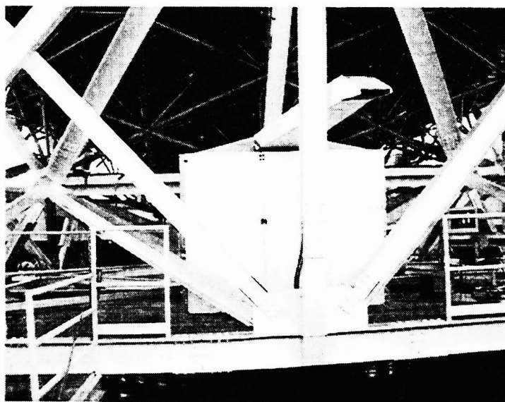
Figure 6: Electronics Bay Enclosure below Primary Mirror
