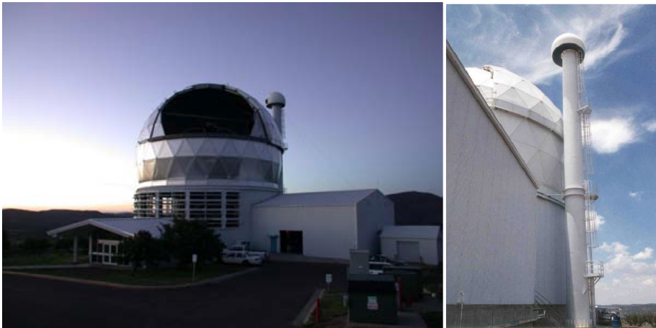
Figure 2 The HET facility (left) [5] and the CCAS tower (right) [16] .
