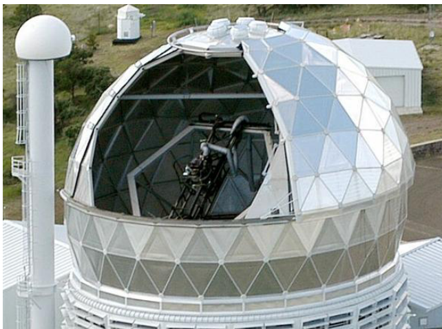
Figure 1. In the photograph at left, the existing PFIP and tracker are visible through the opening in the dome of the HET. The concept drawing at right shows the new PFIP and tracker and also illustrates one of several approaches for mounting VIRUS enclosures on the telescope superstructure.
