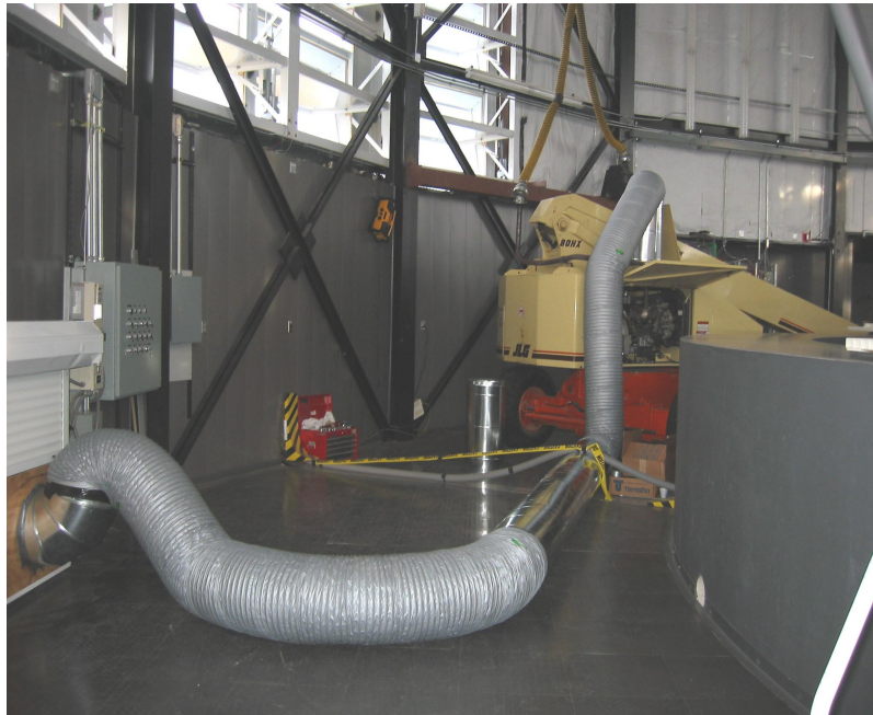
Figure 7: Early operation of JLG ducting
