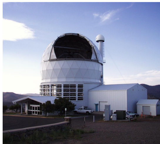
Figure 1: HET at sunset, showing new ring wall louvers.
