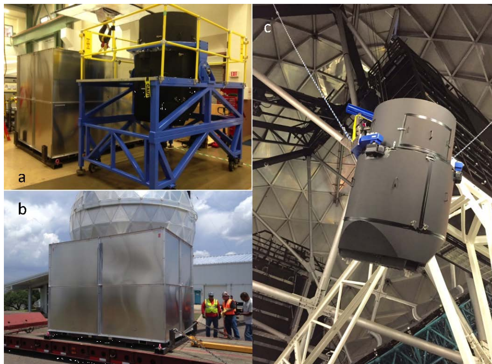
Figure 5: Images of completed HET WFC being transported and installed. (a) WFC in its handling cart next to transportation box; (b) WFC arriving at HET after overnight transportation; (c) WFC mid-air being hoisted into position in the HET tracker.
